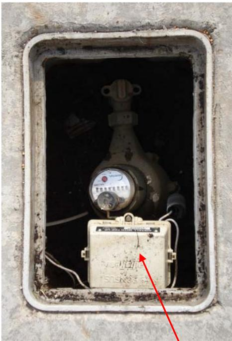
Radio Meter with MXU
